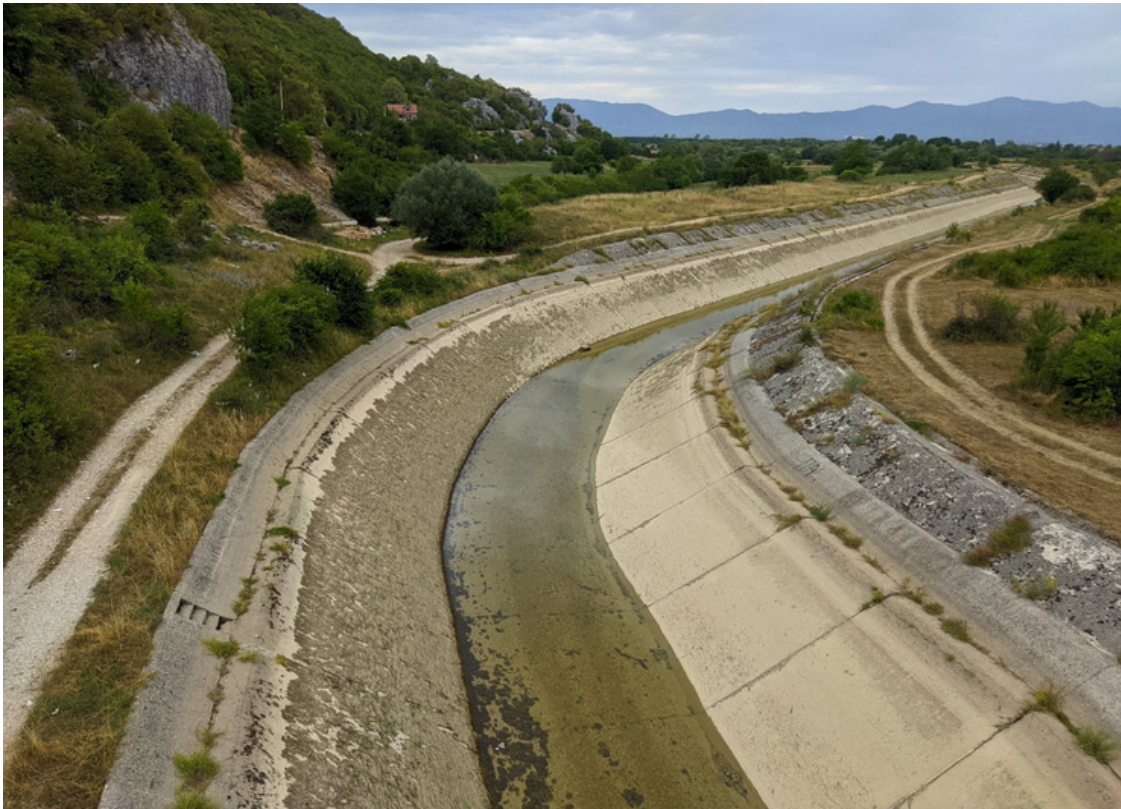
Figure 5. Part of the upper course of the Zeta River canalized for hydropower needs
